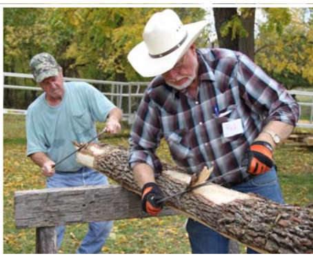
Lee Taylor and Red Pearcy use draw knives to shave bark off a log to be used as the floor of the smoke house.
